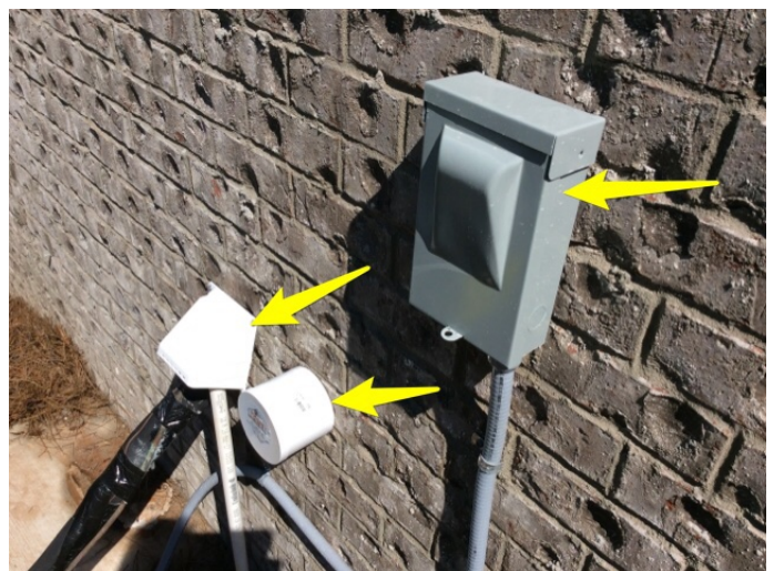
around left side electrical disconnect box, A/C pipe set cover, a...
