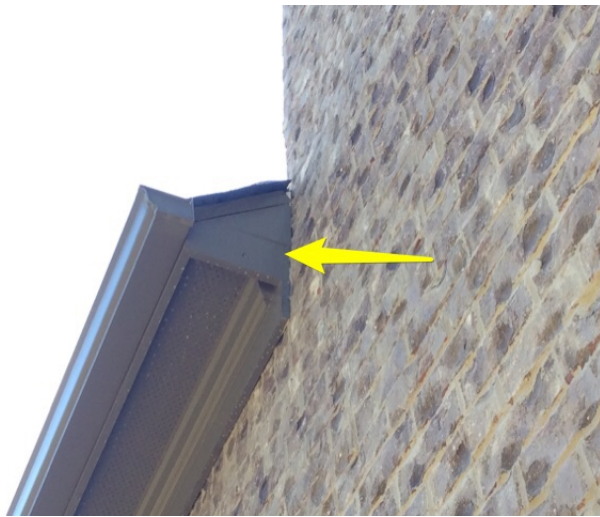
right side soffit end/brick junction
