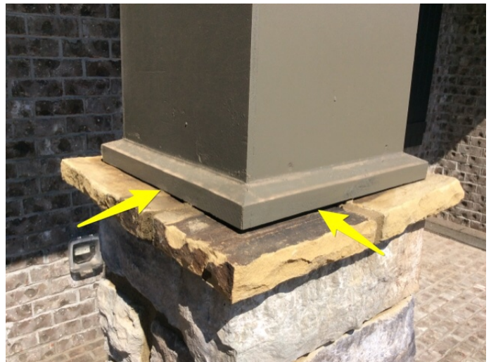
around front porch column base trim/stone junctions
